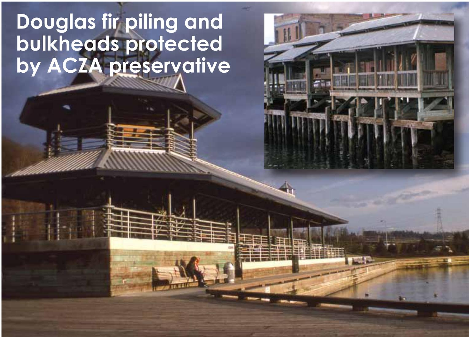
Douglas fir and ACZA is a match made for heavy duty applications. The strength and resilience of Douglas fir, combined with the long-term protection of Ammoniacal Copper Zinc Arsenate (ACZA) preservative, yield a construction material that has been providing reliable service for decades – in utility poles, building poles, foundation piling, bridge girders, roller coasters, and other demanding applications.
