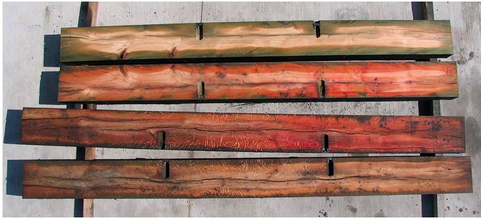
Figure 1. Commercially dual-treated borate (Cellutreat® liquid 50) and copper naphthenate (QNAP®) bridge timbers. Timbers have been rip sawn after borate and plug (BTX®) installation and Boulton treatment, and one half subsequently curcumin sprayed (Smith and Williams 1969) to show the presence of borate (red). For color interpretation of this caption reader should refer online.
