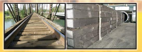
**CONDUCTIVITY.** Tests have indicated that the metallic oxides in ACZA are not conductive. Regardless of the test method used, a bigger factor than wood species or preservative was moisture, which affects all types of treated wood crossties.
