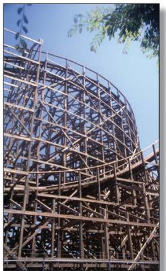
wood exposed by cutting or drilling should be adequately field-treated. Avoid removing the outer shell of wood where treatment is heaviest and resistance greatest. It is recommended that all structures be prefabricated before treatment; minimize problems by specifying framing and boring before treatment whenever possible.
